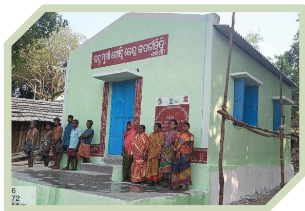
MPCH Building at Kadalidih under CBM
