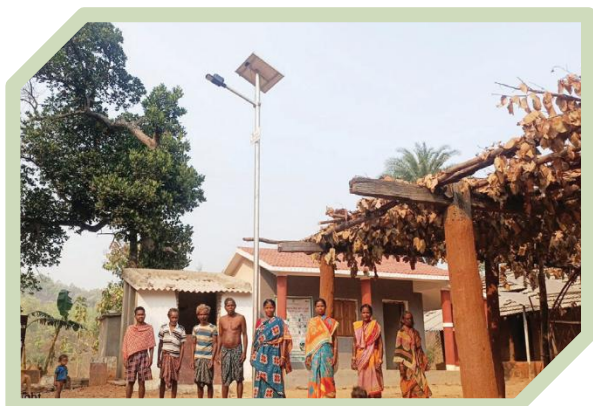
Installation of Street Light at Kaladu
